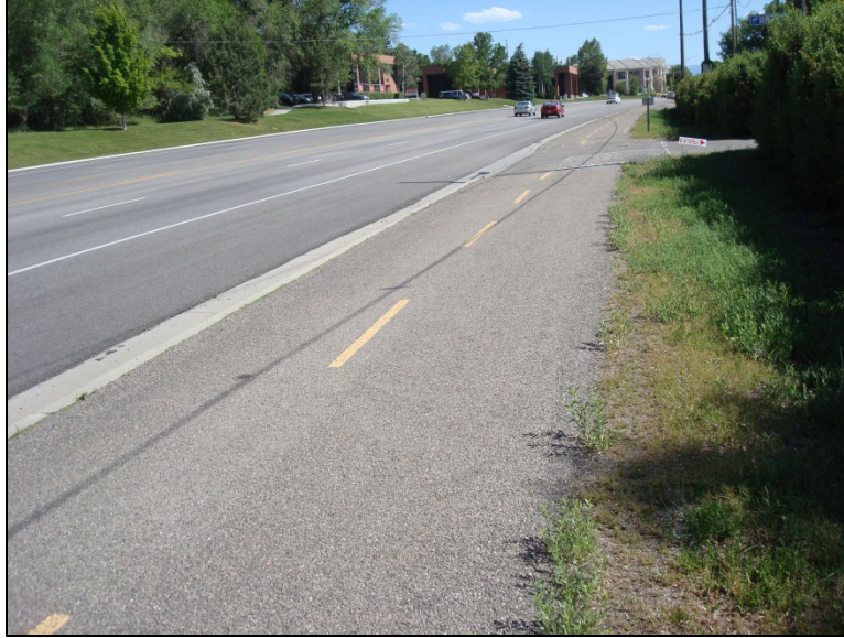
Figure 5-29: Southbound view of the shared use path on University Avenue at Marrcrest East, Provo (photo taken by Chris Haskell, 2015).
