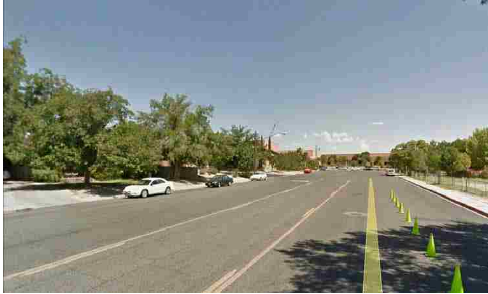
Figure 5-51: View of 400 South at 650 East, St. George (Google Earth, 2015).
