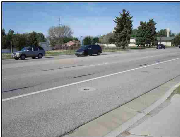
Figure 5-15: View of 10600 South at 1450 West, South Jordan (photo taken by Chris Haskell, 2015).
