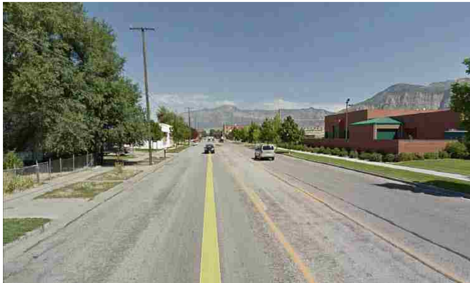
Figure 5-54: View of Lincoln Ave at 2125 South, Ogden (Google Earth, 2015).
