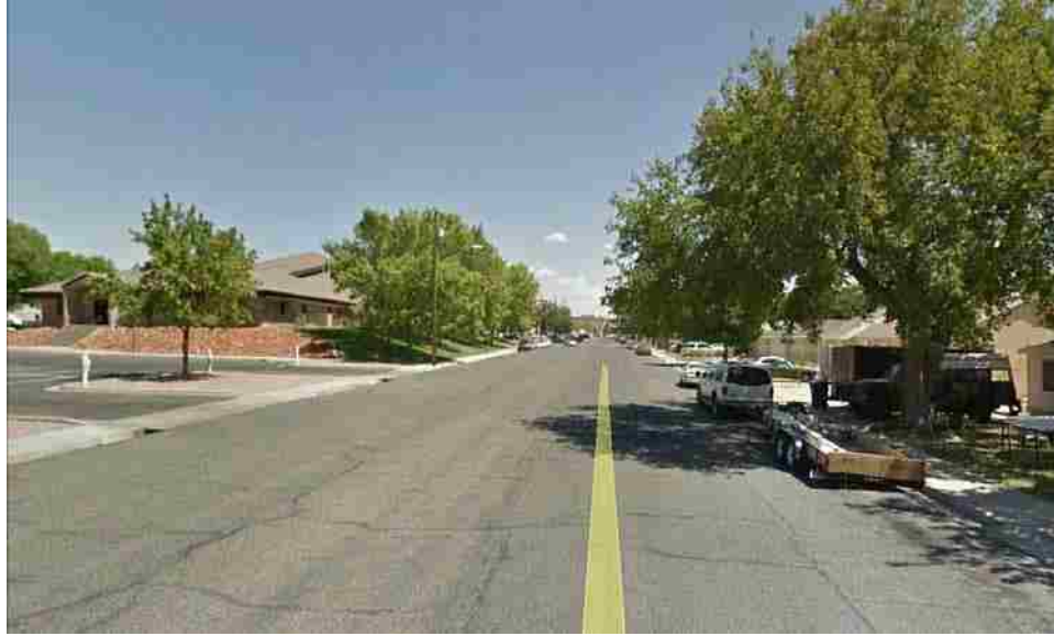
Figure 5-50: View of 300 South at 650 East, St. George (Google Earth, 2015).
