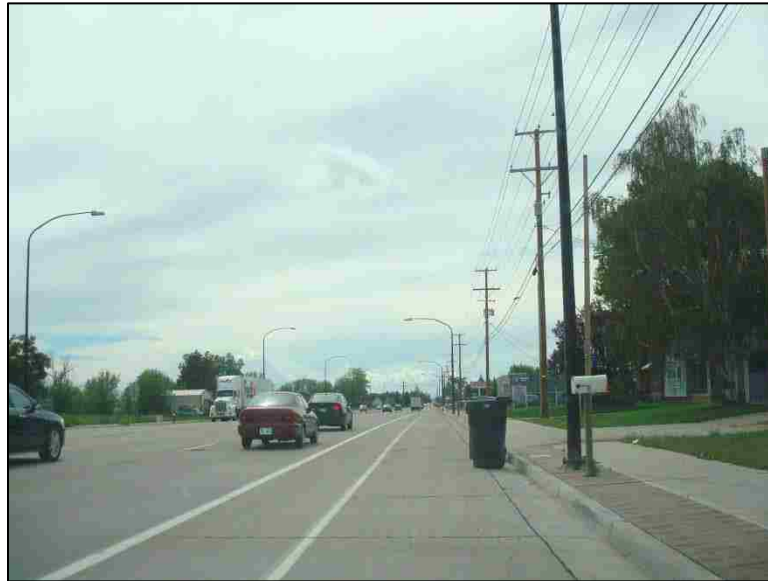
Figure 5-4: Westbound view of the bike lane on 1700 South, Syracuse (photo taken by Chris Haskell, 2015).
