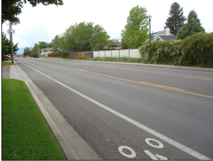
Figure 5-26: View of Orem Boulevard at 250 North, Orem (photo taken by Chris Haskell, 2015).
