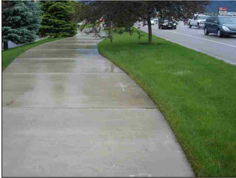
Figure 5-21: Eastbound view of shared use path on 800 North at 480 West, Orem (photo taken by Chris Haskell, 2015).
