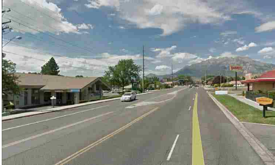
Figure 5-32: View of Freedom Boulevard at 1720 North, Provo (Google Earth, 2015).
