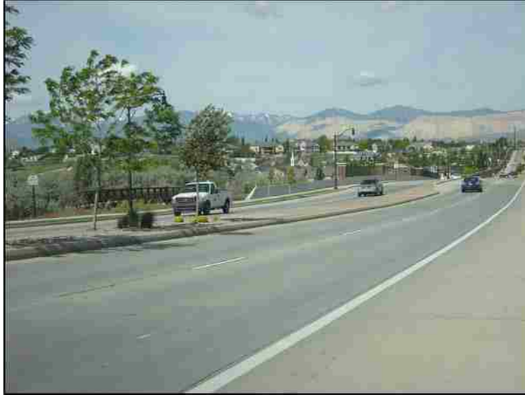
Figure 5-17: View of 11400 South at 1250 West, South Jordan (photo taken by Chris Haskell, 2015).
